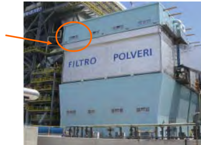
Torrevaldaliga North Fabric Filter Unit 4
